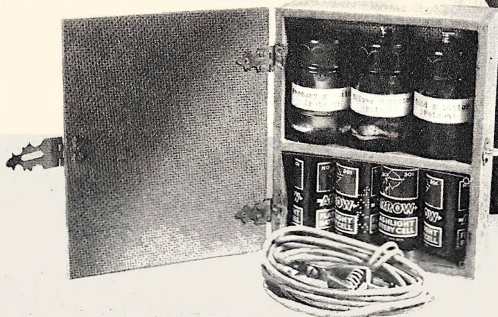
The compact carrying case (above) holds everything you need for electroplating with gold or silver. On opening the lid of the case (left), the plating solutions and current source are readily available. Left, above—Wiring diagram showing how change of circuit can be made to increase voltage delivered by the batteries.
