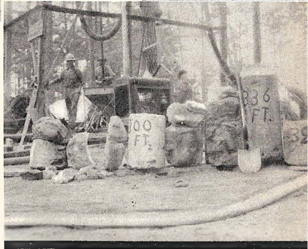
Left—Preparing the outer casing of a well. When in an upright position over the well hole, these huge pipes will be welded together electrically so that they will form one continuous cylinder reaching to the well bottom. Below—Cores of various kinds of formations encountered during the digging of a deep-well. The numerals indicate depths at which formations were located.
