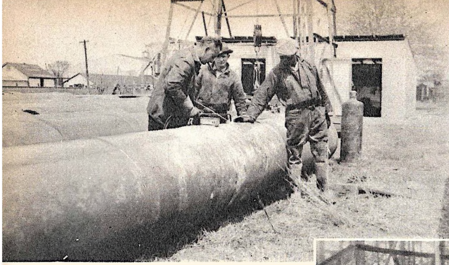
Left—Preparing the outer casing of a well. When in an upright position over the well hole, these huge pipes will be welded together electrically so that they will form one continuous cylinder reaching to the well bottom. Below—Cores of various kinds of formations encountered during the digging of a deep-well. The numerals indicate depths at which formations were located.
