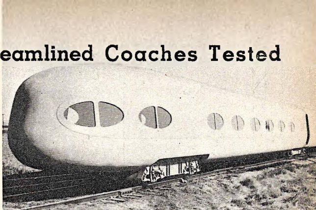
Featuring pendulum-type supports, these two new streamlined railway coaches are mounted on only three trucks. The special mounting enables the coaches to bank when rounding curves.
