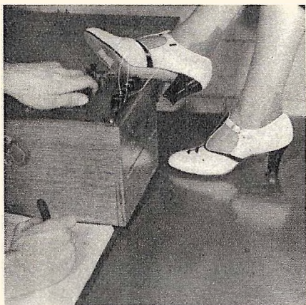
Inserted between the soles of shoes, as shown above, fibrous glass effectively insulates the feet against heat and cold. Left—Checking the temperature within an insulated shoe with a thermocouple device.
